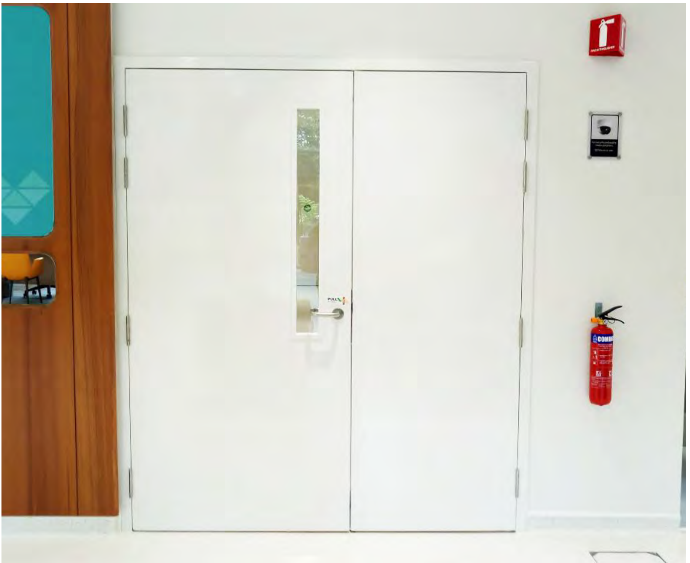
1 HR FIRE RATED DOUBLE LEAF TIMBER DOOR
