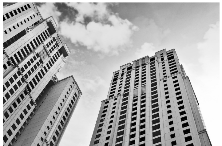
HOUSING (INCLUDING BUT NOT LIMITED TO HDB, CONDOMINIUM AND APARTMENT)
