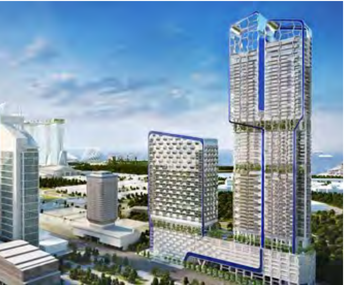
UIC Redevelopment (V on Shenton)
